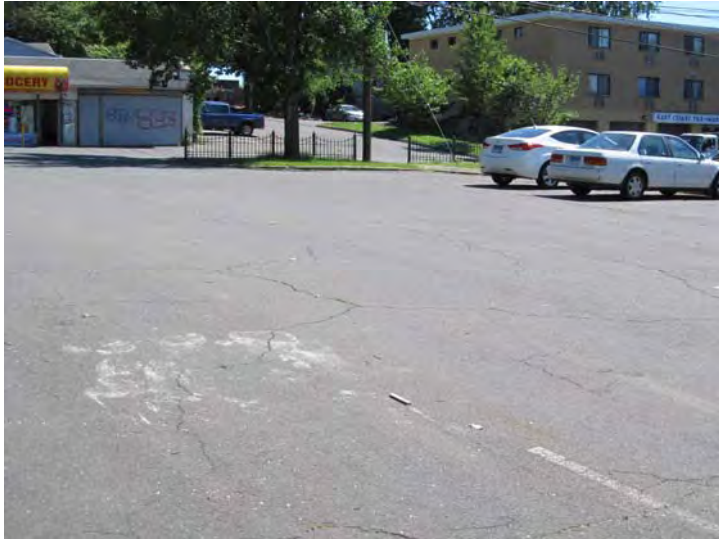
Asphalt paving in need of crackfilling, sealcoating, and striping in the near-term
