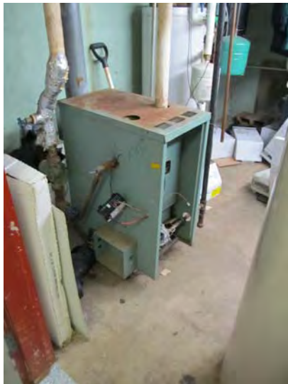
Boiler at maintenance shop is operable but has surpassed its expected useful service life
