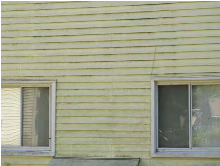
Significant dirt/organic growth widespread on vinyl sided exterior wall surfaces
