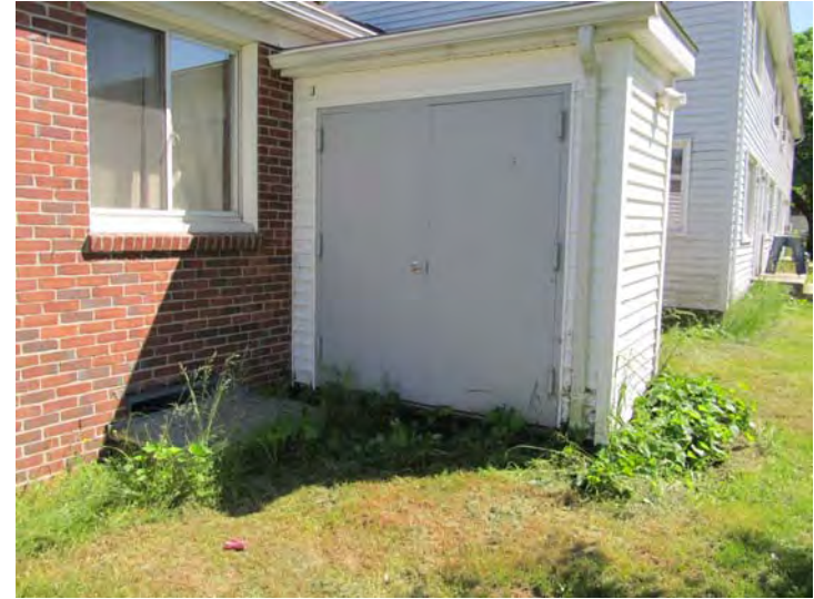
Typical 'doghouse' at residential building housing mechanical equipment – 'Doghouse' construction completed as part of unit mechanical system upgrades in recent years
