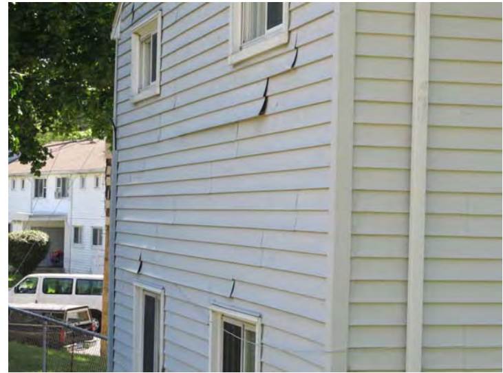
Loose vinyl siding seams noted at several locations
