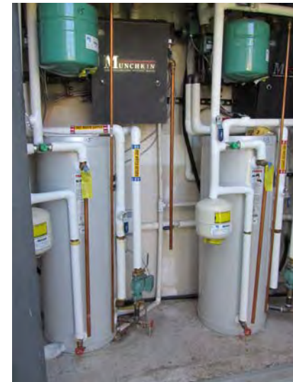
Each unit has a recently installed wall-mounted boiler and a freestanding, indirect-fired, domestic hot water tank
