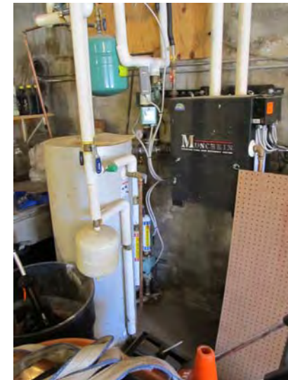
Boiler and domestic hot water generation equipment serving maintenance garage were upgraded in recent years
